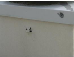
Apply compatible roofing cement/sealant.
