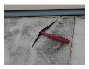
Clean and apply compatible roofing cement/sealant.
