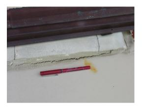
Remove old sealant, clean and apply compatible roofing cement/sealant.
